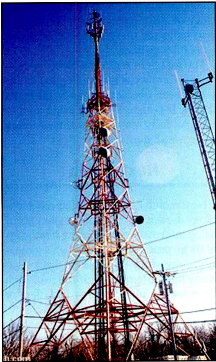
The antenna for the United States' first commercial FM broadcaster was located on Mt. Asnebumskit near Paxton, Massachusetts, and was completed in 1938. The station operated as WIXOJ on 43 MHz at 50,000 watts until the FCC ordered all FM broadcasters to move to the current FM band in 1945. The tower remains in operation to this day. It's 400 feet high and sits at 1,400 feet above sea level, providing a very good signal to the Boston area. The transmitter was originally linked to the studio 42 miles away by a repeater transmitter operating at 133 MHz. After 1945 the station converted its transmitter and antenna to the higher frequencies and operated under the callsign WAAB, which it later changed to WAAF in 1967. (Photo courtesy www.tybush.com )
